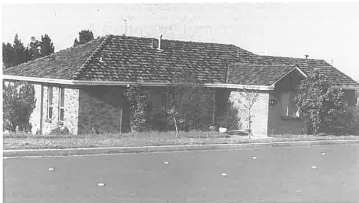
We pitched the new roof.
